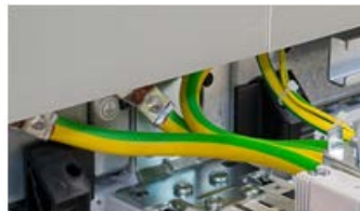
Figure 6-48 Example: Protective conductor with GREEN-AND-YELLOW insulation
