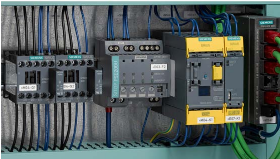
Figure 6-61 Example: Reference designations on various items of equipment in the control panel
