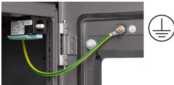
Figure 6-67 Example: Marking with the symbol IEC 60417-5019
