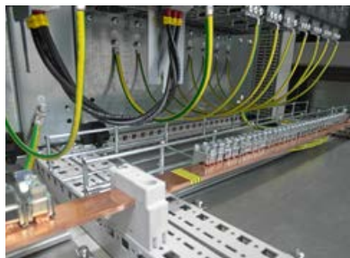
Figure 6-68 Example: Marking with GREEN-AND-YELLOW at the end of the protective conductor busbar
